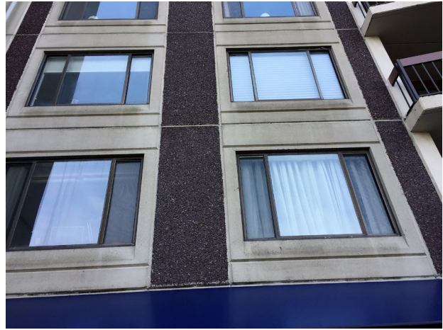
Photograph 9 – Example of the exterior wall concrete panels.
