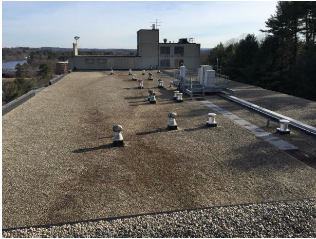
Photograph 8 – View of the main roof.
