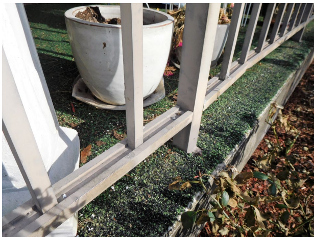
Photograph 10 – Example of typical aluminum balcony railing components.
