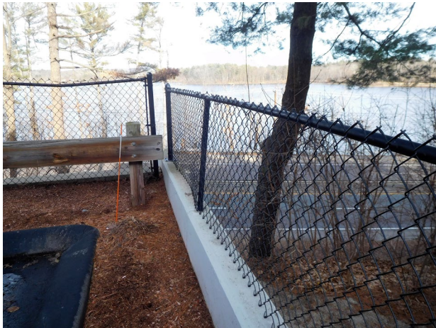
Photograph 2 – View of the chain link fence.
