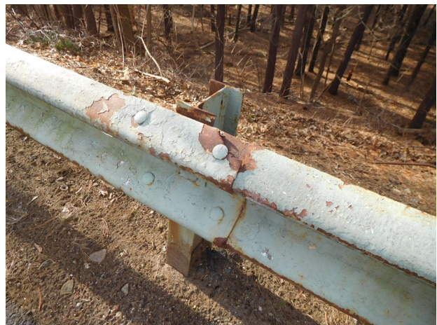
Photograph 5 – Example of the steel guardrail.
