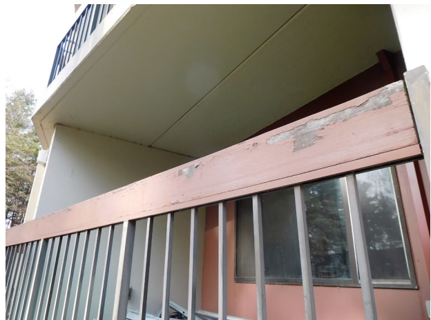
Photograph 11 – Example of a typical balcony wood top rail.
